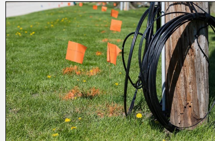
Figure 6: Example of Underground Utility Locating
